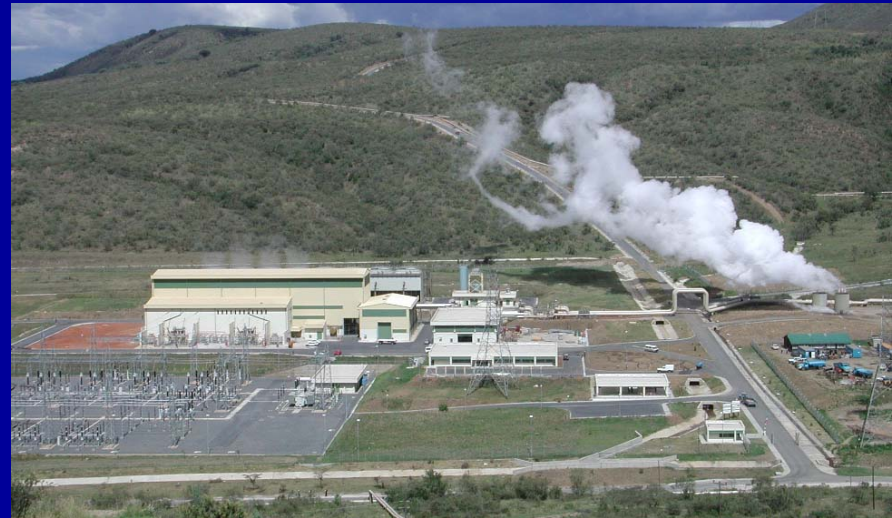
Olkaria II Power Plant 70MW / 35 MWe under construction
